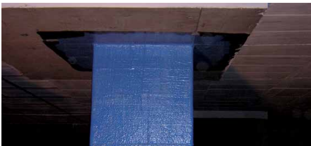
Load Carrying Capacity Enhancement
