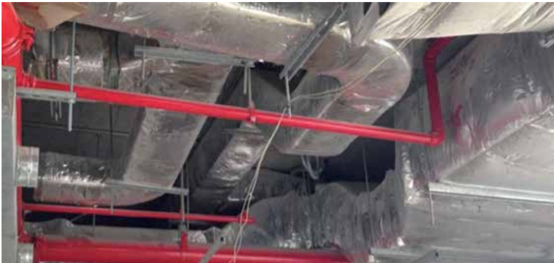
Installation Of Fire Fighting Systems
