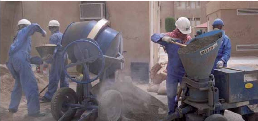
Mixing Concrete Admixtures
