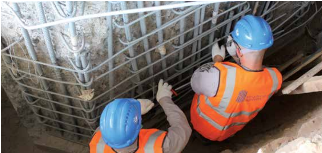
Reinforcing Steel Replacement
