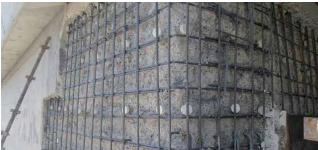
Concrete Repair and Protection
