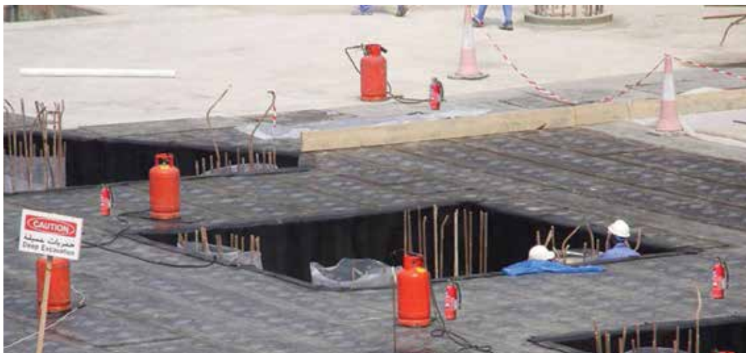
Bituminous On Raft Foundation
