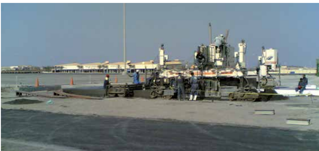
Concrete Paving Using Wirtgen SP 500
