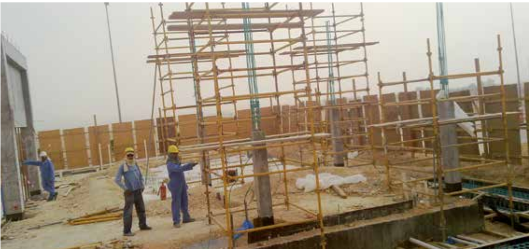
Reinforced Concrete Works
