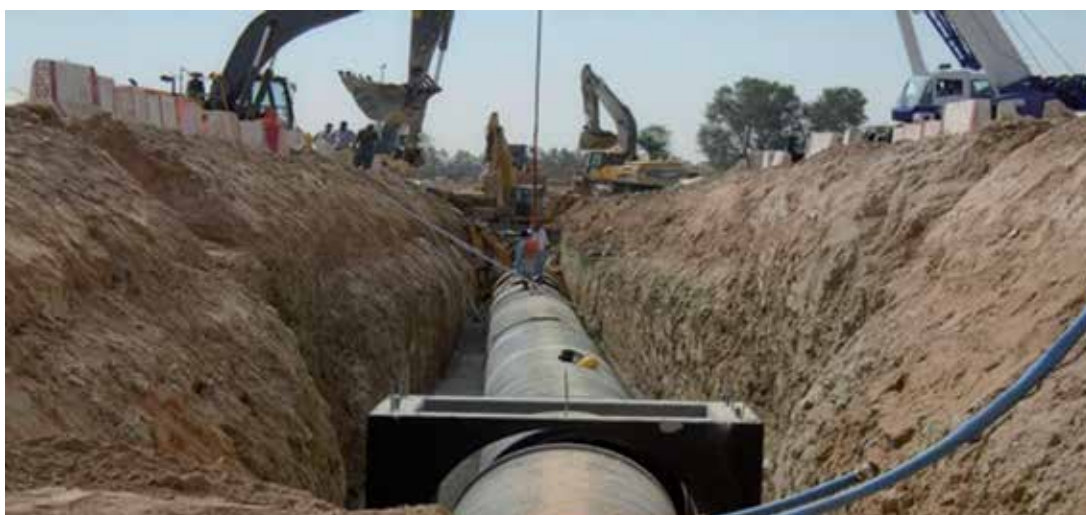
Infrastructure Work For Storm Water Drainage & Sewage
