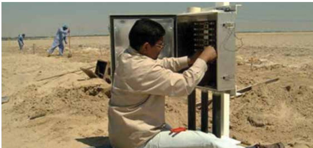
Cathodic Protection Installation & Commissioning
