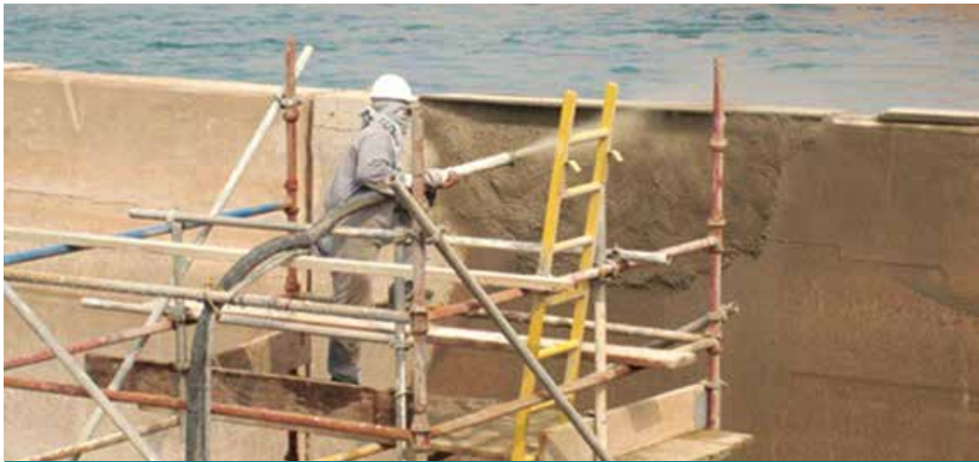
Retaining Wall Concrete Repair
