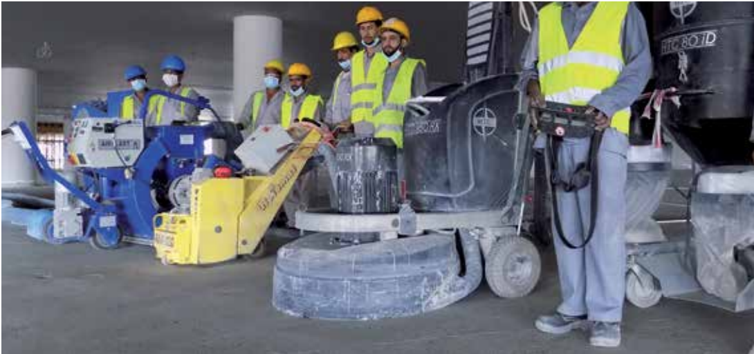
Floor Surface Preparation
