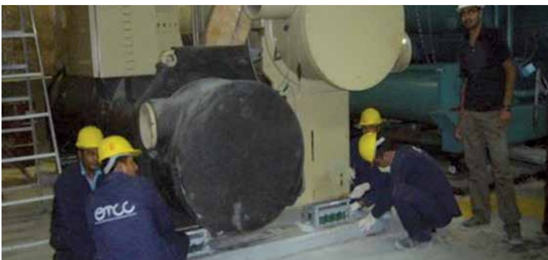
Electromechanical Equipment Commissioning
