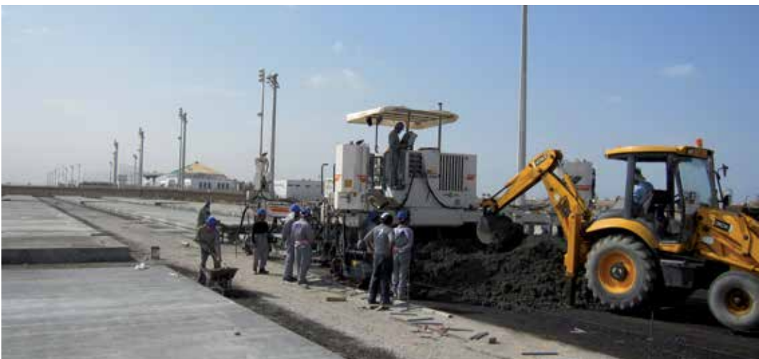
Concrete Casting For Airport Apron Slab
