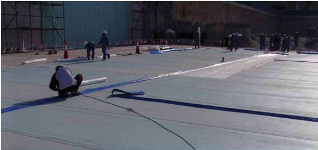
Water Stop Welding
