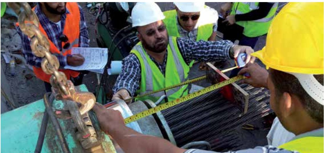
Strands Threading Using Pushing Machine
