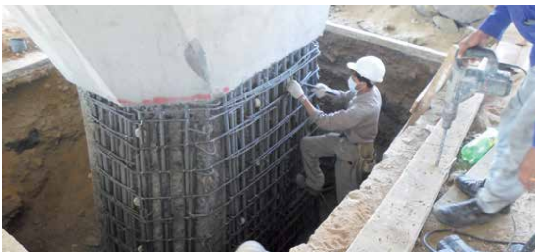
Bridge Column Repair
