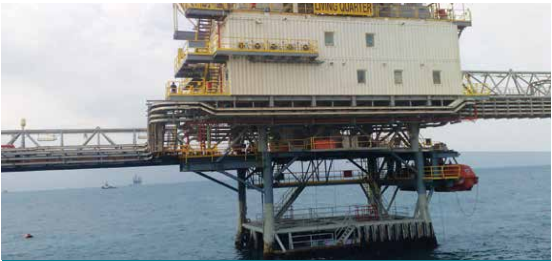
Cathodic Protection For Platforms
