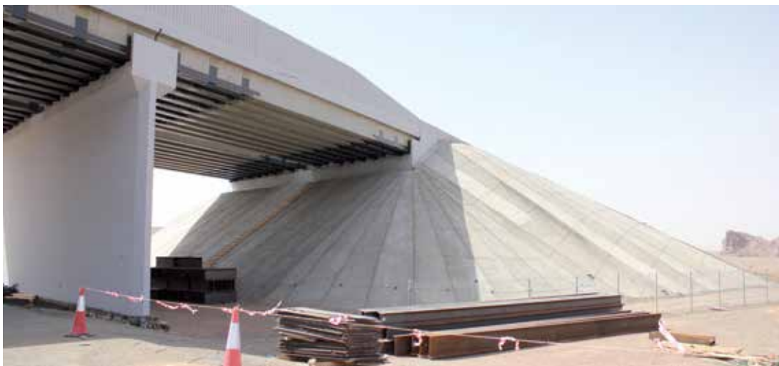
Bridge Repair - CFRP
