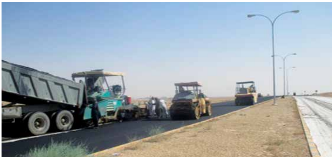
Road Construction & Paving
