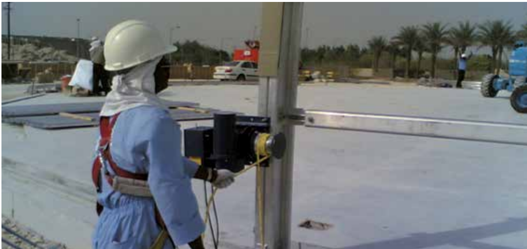
Structural Framing & Cladding Works
