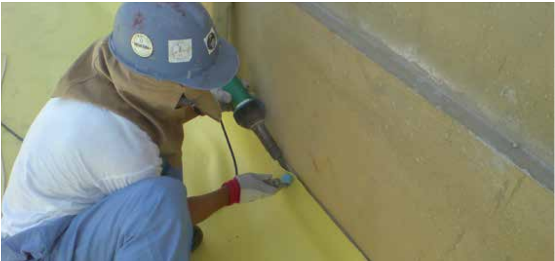
PVC Hot Air Welding
