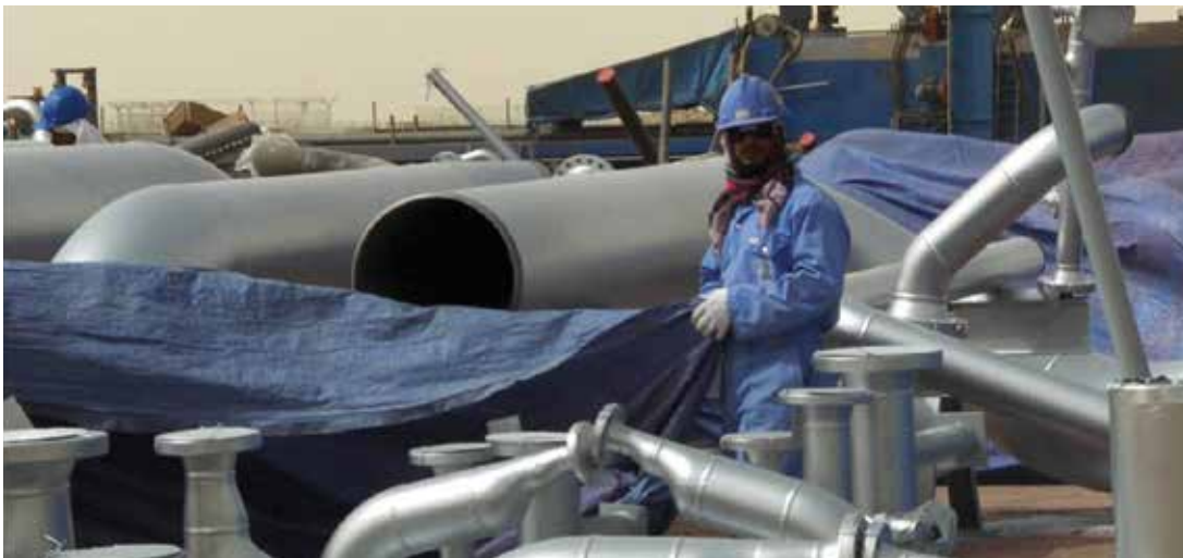
Steel Protective Painting
