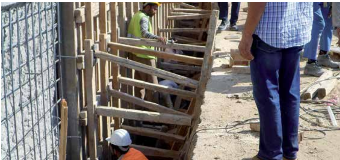
Form & Pump, Concrete Repair
