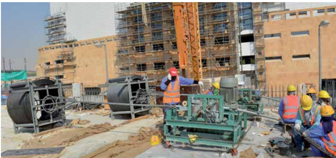
Tendon Stressing Operation
