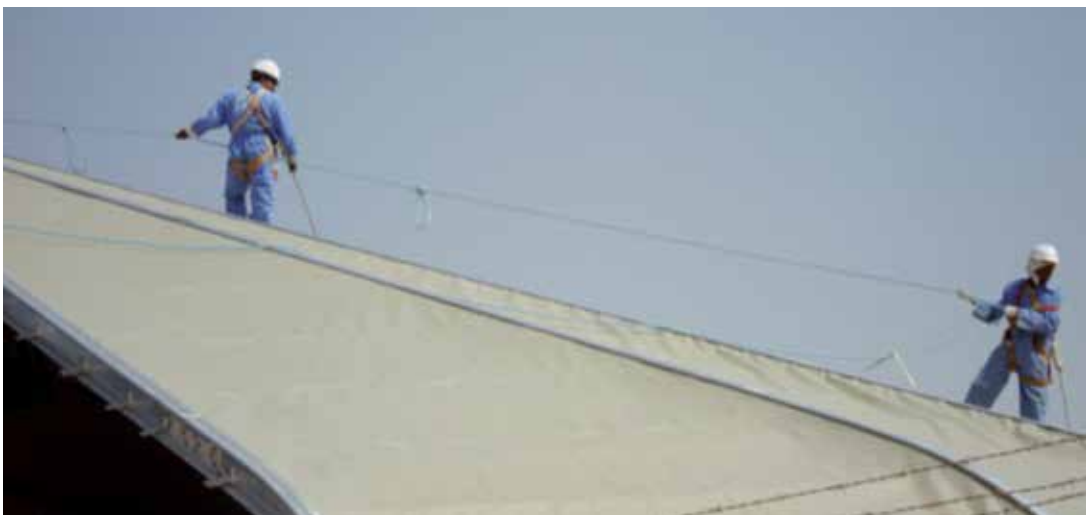
Sloped Roof With Insulated Panels
