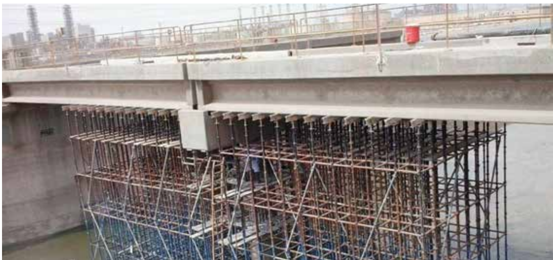
Bridge Structural Repair
