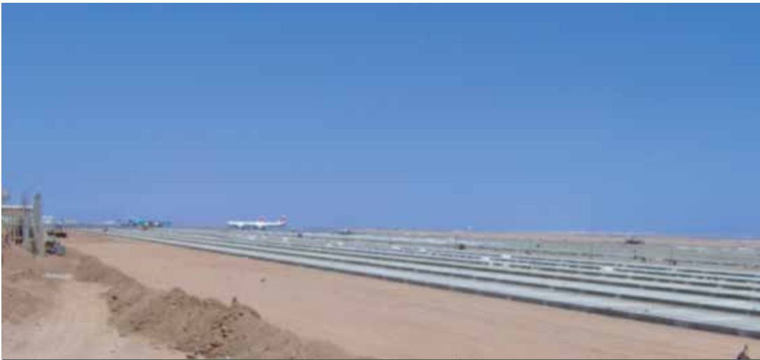
Concrete Paving For Airport Apron Slabs
