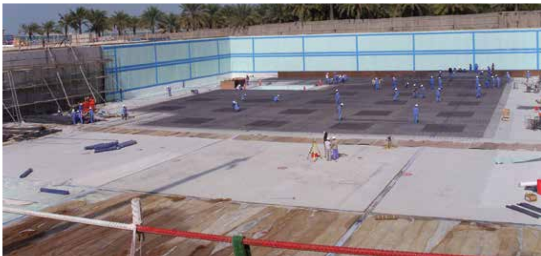
Underground PVC Compartment
