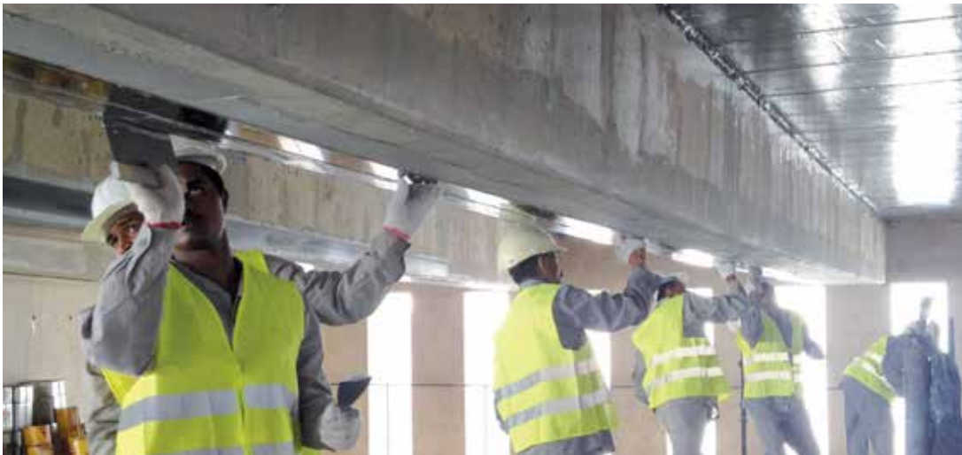
CFRP Slab Reinforcement
