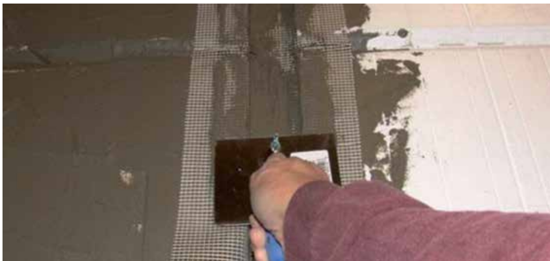
Basecoat & Mesh Detailing
