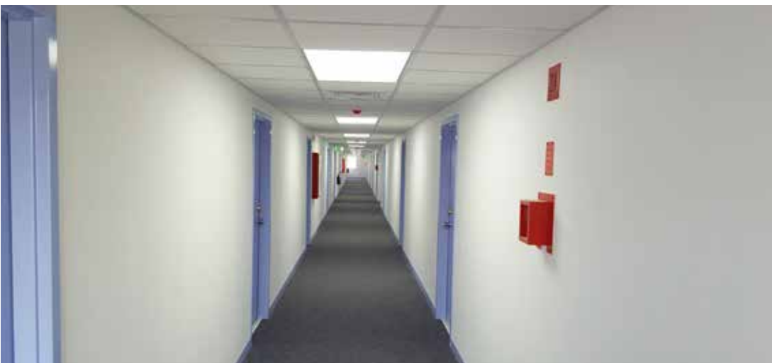
Acoustical Ceiling, Fire Alarm & Fire Fighting Works
