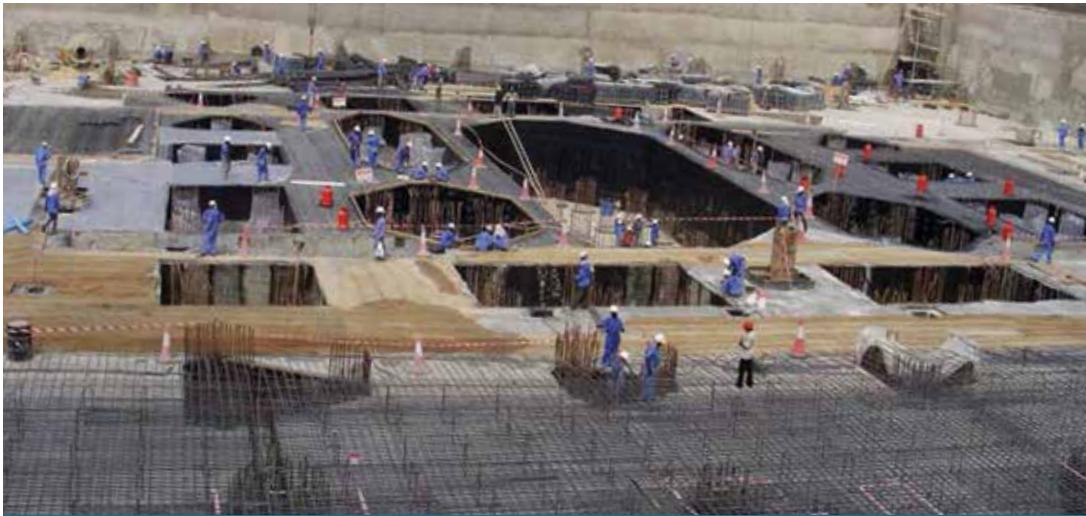
Substructure Bituminous Waterproofing
