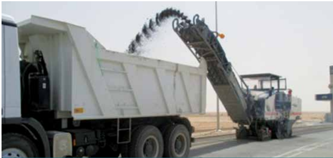
Milling & Asphalt Resurfacing
